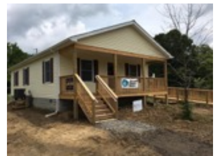
Several organizations partnered on funding construction of this home in Fayette County after the June 2016 flood.
